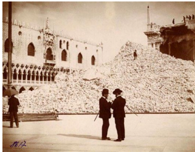
Piazza San Marco in Venice after the collapse of the Campanile (1902).
